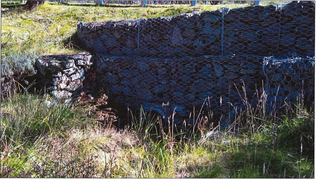
Figure 13: Existing discharge point of stormwater below Friday Drive (Source: Department inspection)
