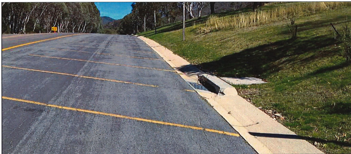
Figure 12: Existing stormwater pit on Friday Drive (Source: Department inspection)
