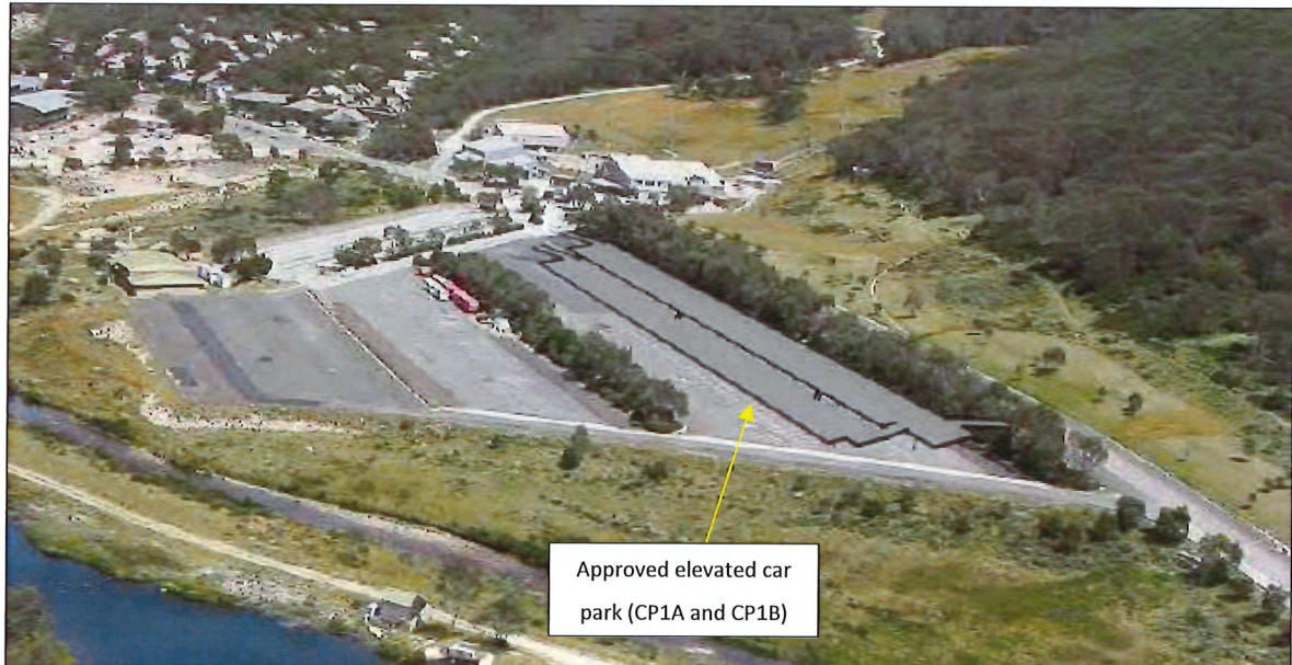
Figure 4: Photomontage of proposal in context of existing car park (Source: Applicant's documentation)
